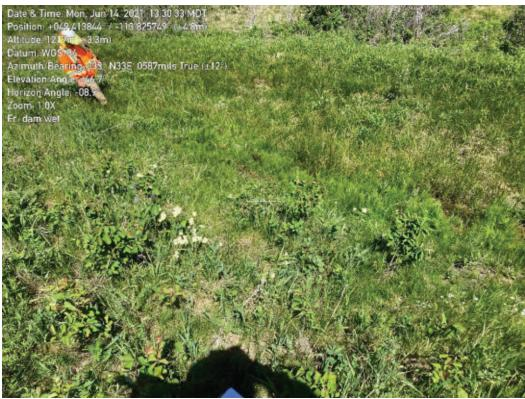
Photograph 2-9 Dam downstream slope (natural section), where soft and wet ground condition as well as standing water were observed, looking down
