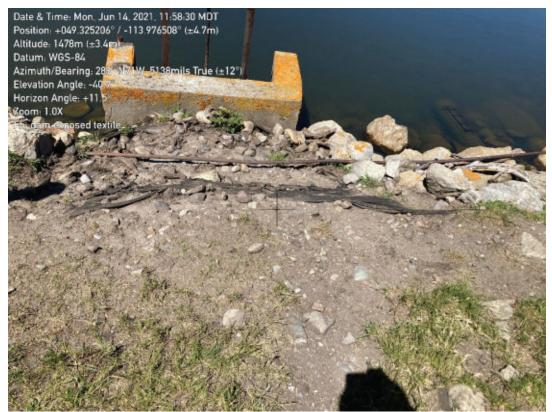
Photograph 5-15 Exposed geotextile behind inlet concrete headwall
