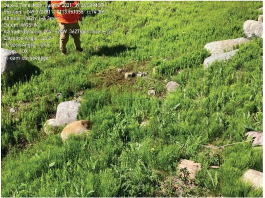
Photograph 1-16 soft and wet ground at the downstream slope toe
