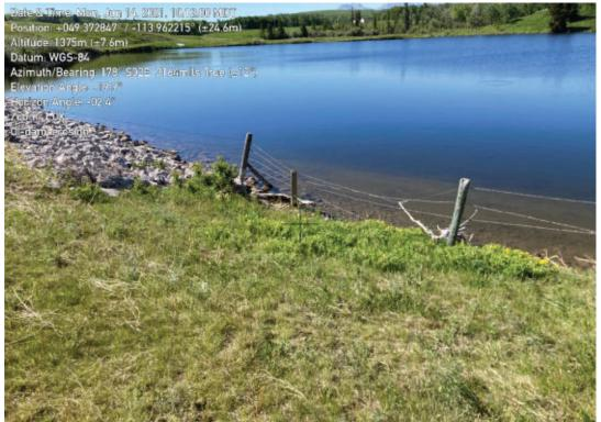
Photograph 1-4 Eroded bank and fallen fences, at the north end of the dam's upstream slope, adjacent to the abutment
