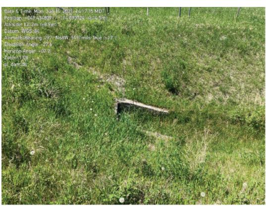
Photograph 3-3 Dam downstream slope and outlet headwall
