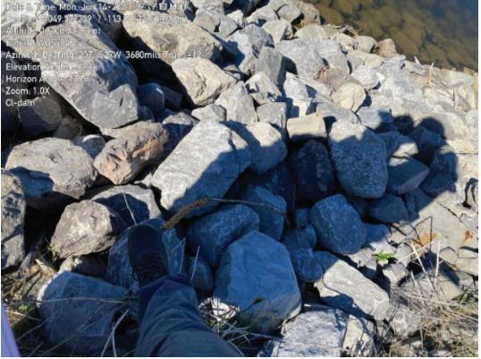
Photograph 1-6 Riprap sizes compared to 9.5-size boot
