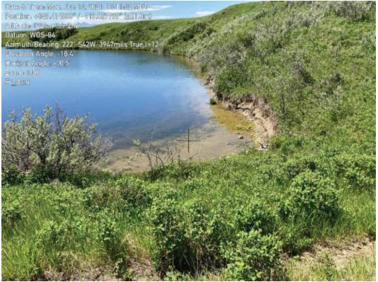
Photograph 2-4 Eroded bank at the north end of the dam upstream slope
