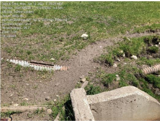
Photograph 5-11 Exposed CSP outlet culvert
