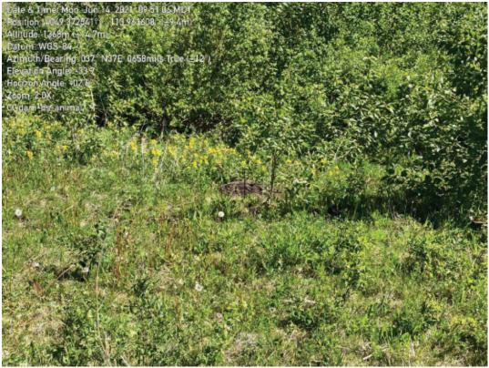
Photograph 1-13 Animal establishment observed on downstream slope
