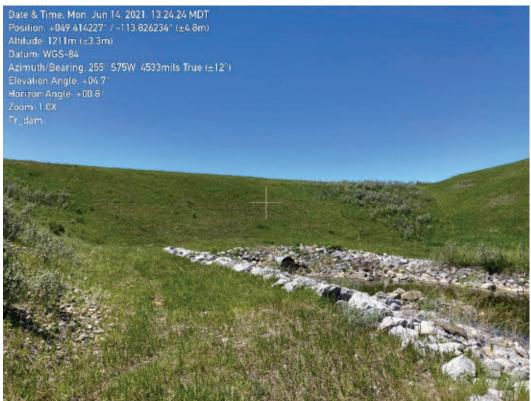
Photograph 2-7 Dam downstream slope (engineered section), looking up, including low level outlet
