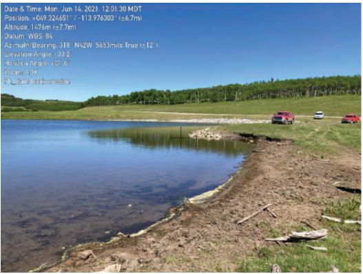
Photograph 5-4 Bank erosion at the junction of the dam and the spillway, facing northwest
