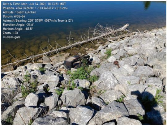
Photograph 1-5 Riprap and inlet control valve on upstream slope
